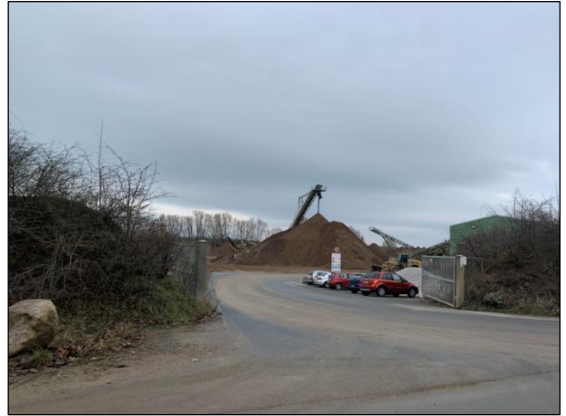
IO-31 Froser Str. 1-2, Reinstedt (Bauschuttrecycling Reinstedt GmbH & Co. KG)
