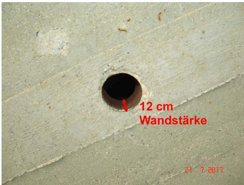
2017H 29 - TW-U LINKS - 5M VOR BWE - HOHLKASTENBODEN 12 CM
