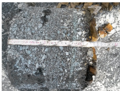
Foto 1: Asphalt Bohrkern (Dicke 23 cm)
