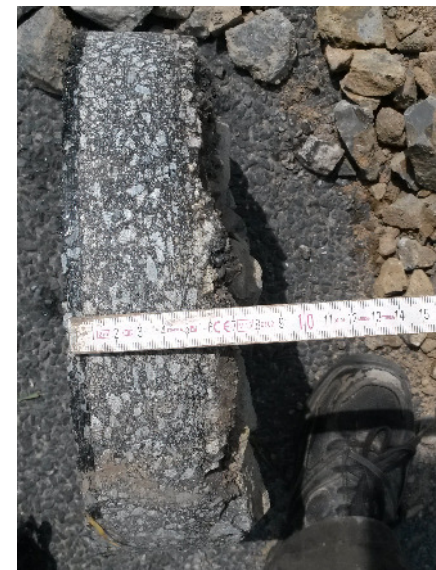
Foto 1: Asphalt Bohrkern (Dicke 1 + 5 = 6 cm)
