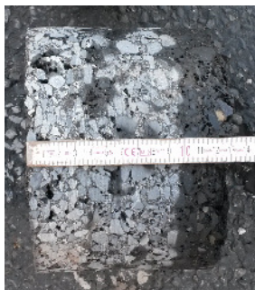
Foto 1: Asphalt Bohrkern (Dicke 13,5 cm)
