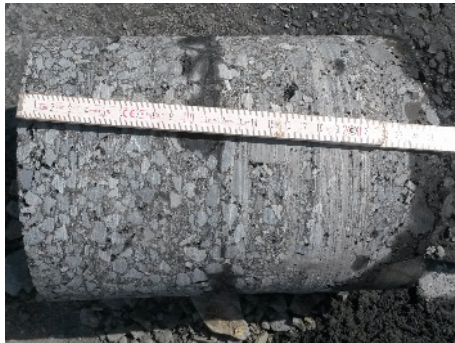
Foto 1: Asphalt Bohrkern, 3-lagig (Dicke 26 cm)
