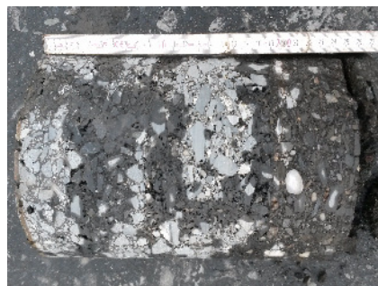
Foto 1: Asphalt Bohrkern (Dicke 25 cm)
