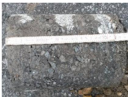
Foto 1: Asphalt Bohrkern (Dicke 23 cm)
