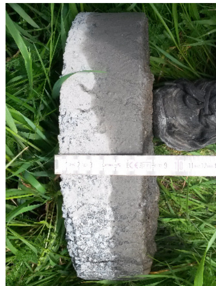
Foto 1: Asphalt Bohrkern (Dicke 1 + 6 = 7 cm)
