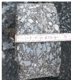
Foto 2: Asphalt Bohrkern (Dicke 9 cm)
