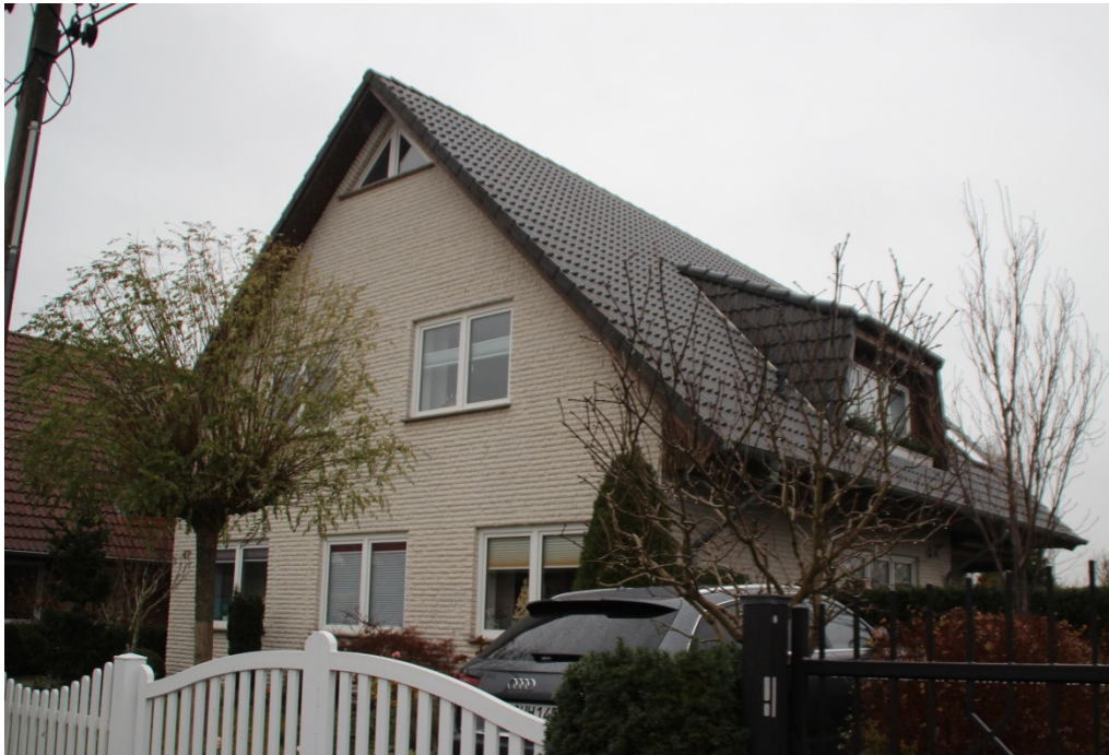
IP BH: Whs. Neue Straße 47, Plate
