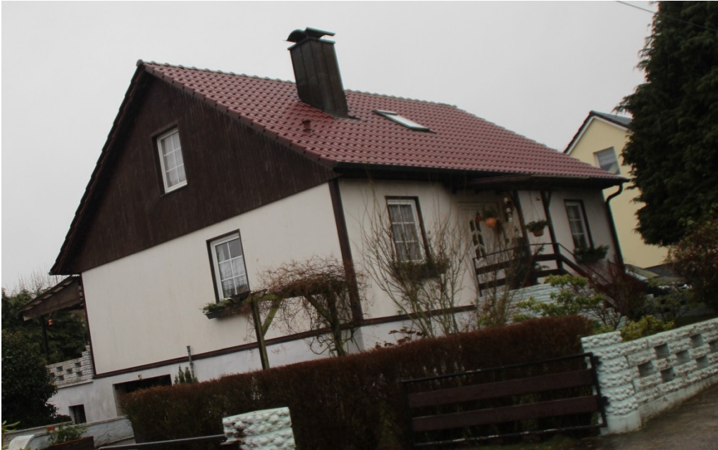
IP CO: Whs. Neue Straße 3c, Plate
