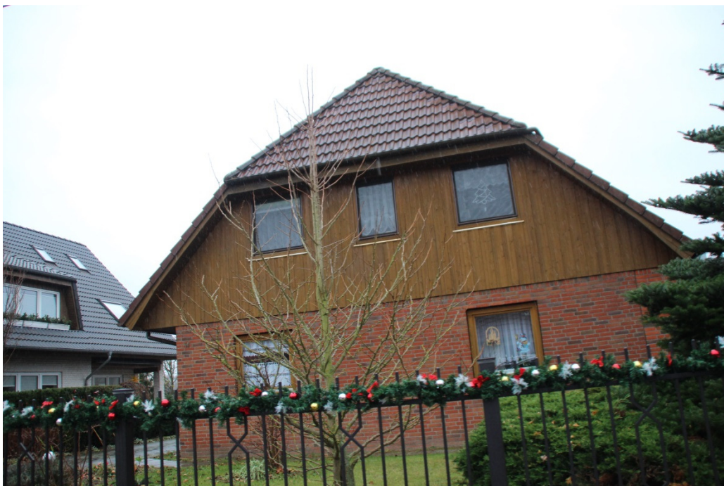
IP BE: Whs. Neue Straße 46, Plate
