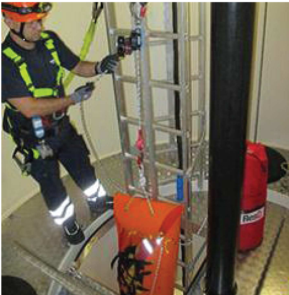
Figure 7.22: Guide the person during lowering when the descent unit is used
