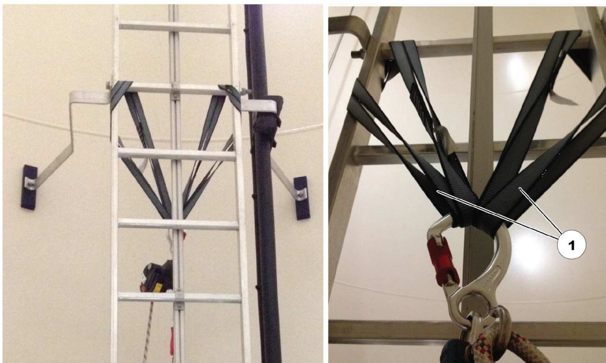
Figure 7.21: Attach the descent unit to the ladder with 2 slings
