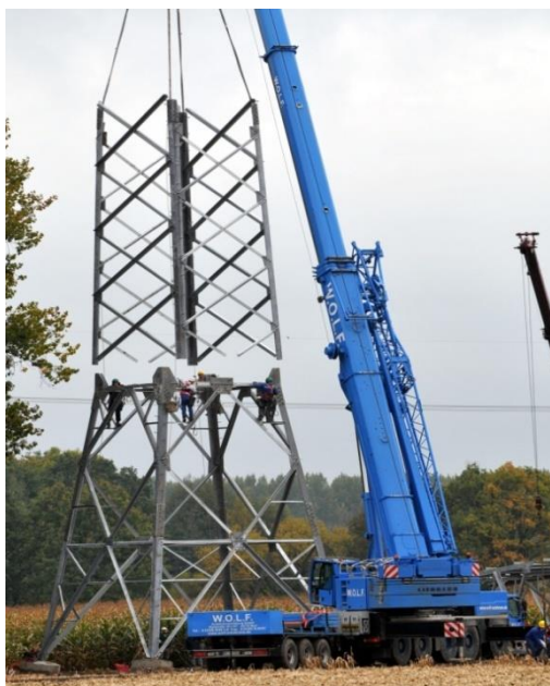
Abb. 6: Mastmontage (Stocken)
